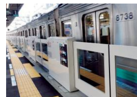
Platform screen doors at Saginuma Station, Den-en-toshi Line
